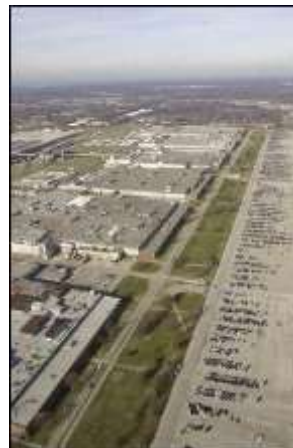
2003 aerial photo of Appliance Park.
